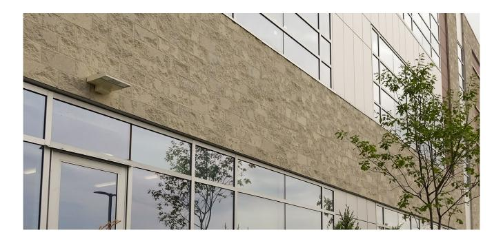
"The Trattino units are a combination of split-face and ground face," notes Wilhelms. "The units are fractured, then run through a grinding machine that takes the high points off the block. So, you have a very unique combination...a very polished surface as well as a rough recessed cavities in the texture of the block. As sunlight hits the wall it really creates some unique interest and adds a depth to the wall that you don't get often with heavy flat materials."
